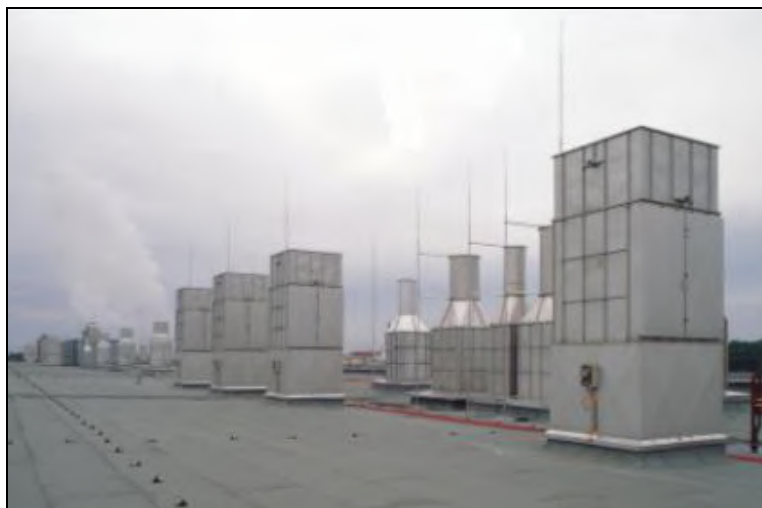
Figure 7.37: Silencers on the paper mill roof
